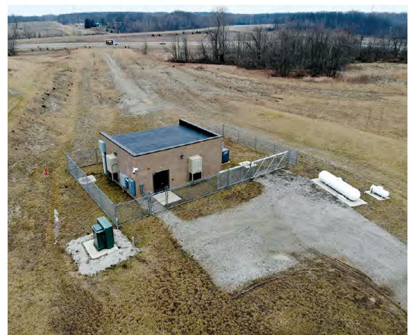
FIGURE 7: Shown is the aerial view of the massive TRC campus. Circled is the US33 Telecom Building shown larger in the right-hand image. It is the termination location for the Phase 1 and Phase 2 cabling backbone infrastructures. (Photos provided with permission and courtesy of TRC Inc.)
