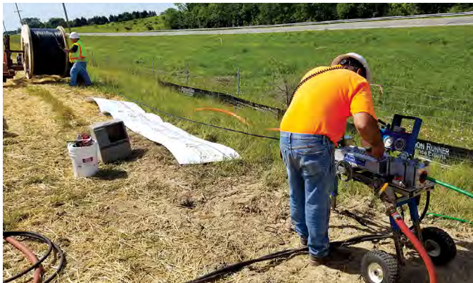
FIGURE 11: The air-jetting equipment set-up.
