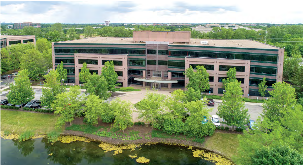
FIGURE 6: The main distribution frame (MDF) is in the MDC, which is a large commercial office building. The MDC occupies the 3rd floor in this building. Image is courtesy of the Union County Chamber of Commerce.
