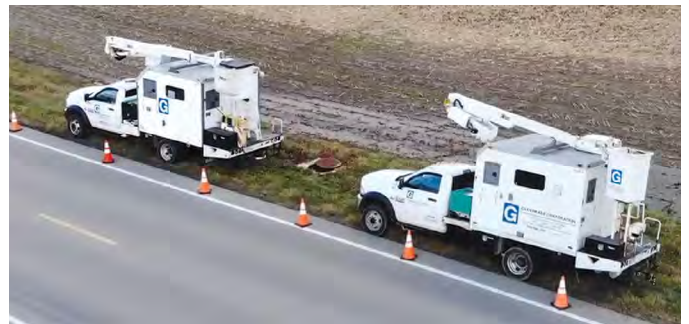
FIGURE 12: Fusion splice trucks.
