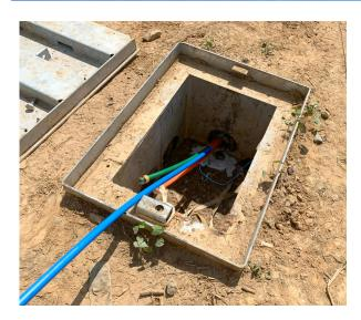
placement of the MicroDuct 16/12 mm with a Condux Gulfstream, and successfully jetted the MicroDuct into the existing 2-inch PVC in a similar method to what would occur in a MicroDuct override. Placement of a 24-count, 7.6mm OD micro fiber optic cable followed with a Plumettaz MiniJet.
