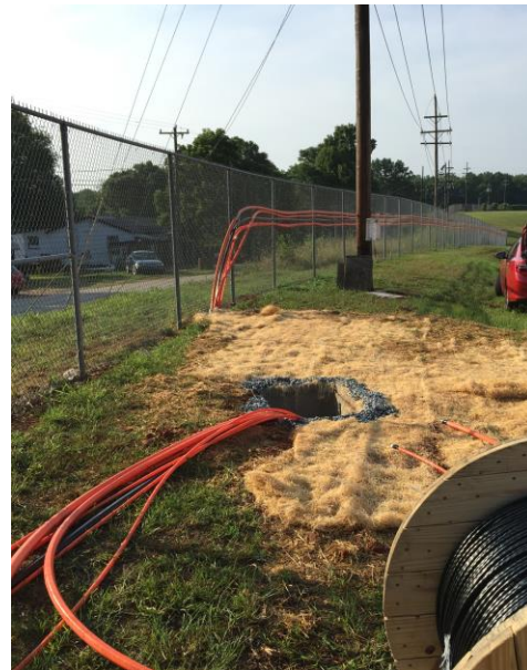
Figure 11. Installation Test Track
