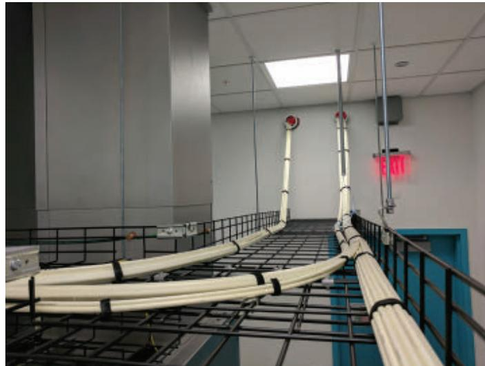
eABF MicroCables can be blown through the Dura-Line MicroDucts anytime and anywhere at a moment’s notice using only two installers, allowing for fiber to be installed into a client suite in an unprecedented 20 minutes.
