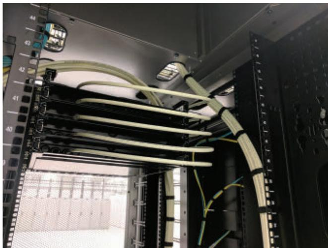
Near termination points, the FuturePath MicroDuct jacket is removed allowing for easy routing and tighter bend radii. Unlike conventional infrastructures, the Dura-Line MicroDuct is a permanent pathway that is installed once and can be reused again and again for the life of the facility.
