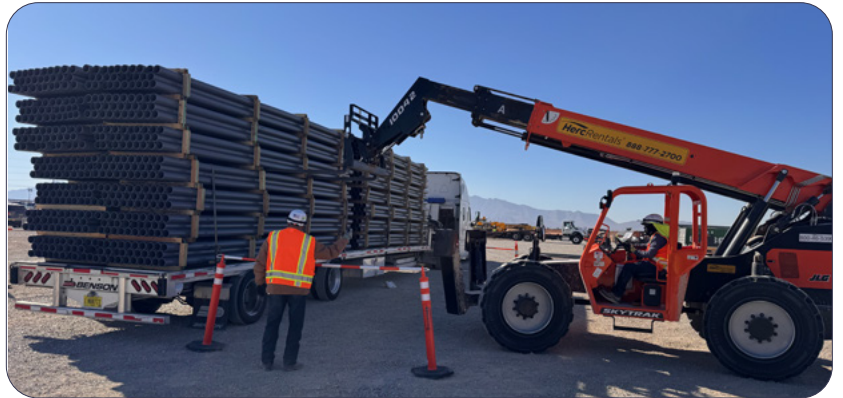
Single-fork truck lifting a bundle of 20' HDPE sticks
