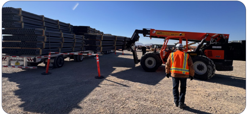
Telehandler lifting a bundle of 20' HDPE sticks
