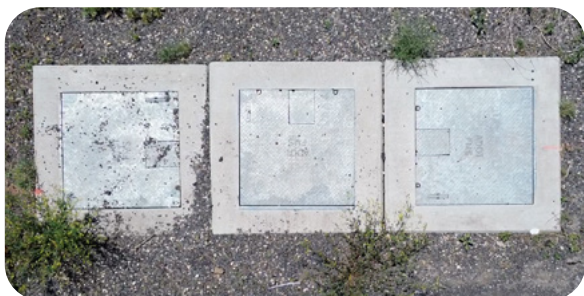
Three vaults in series to accommodate multiple asset owners.
