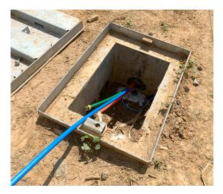
placement of the MicroDuct 16/12 mm with a Condux Gulfstream, and successfully jetted the MicroDuct into the existing 2-inch PVC in a similar method to what would occur in a MicroDuct override. Placement of a 24-count, 7.6mm OD micro fiber optic cable followed with a Plumettaz MiniJet.
