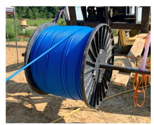
for the second route. Both products are lined with the new Dura-Line SILICORE ULF lining, which decreases friction between the cable jacket and MicroDuct wall, increases jetting distance by up to 25%, and now comes standard on all Dura-Line OSP products.
